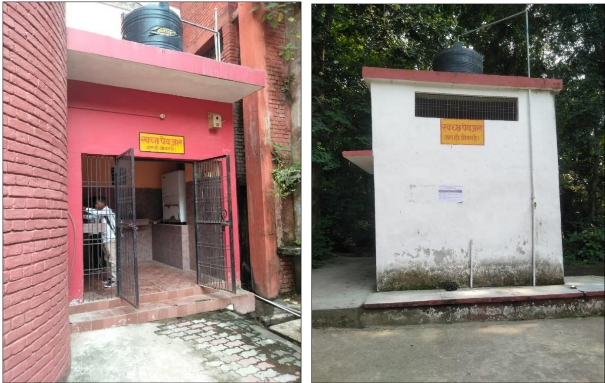
Photographs of Drinking Water Booth with storage tank
